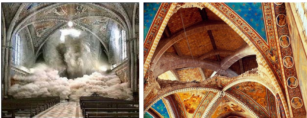
Figure 6.5 Basilica of St. Francis of Assisi collapse of masonry frescoed vaults
