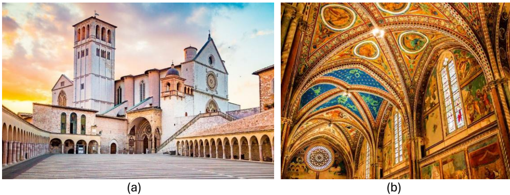
Figure 6.4 Basilica of St. Francis of Assisi (Italy) external view (a), internal view of the vaults (b)
