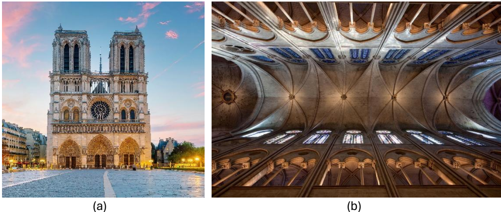
Figure 2.6 Notre-Dame Cathedral, Paris (France) external view (a), internal view of the six-part ribbed vaults (b)
